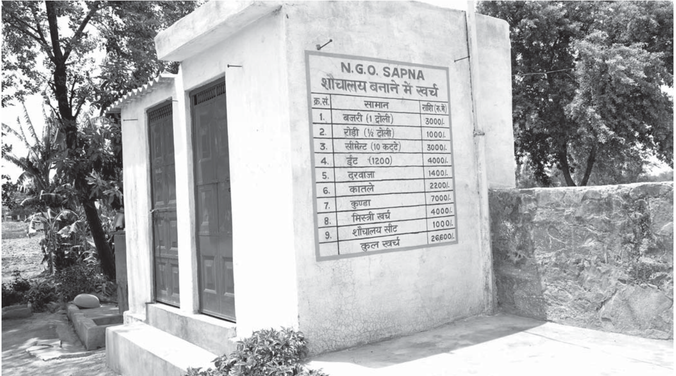
Toilet constructed in model village Kaduki
